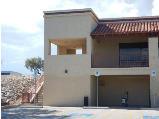
Two railings are visible at the stairs and at the balcony.
